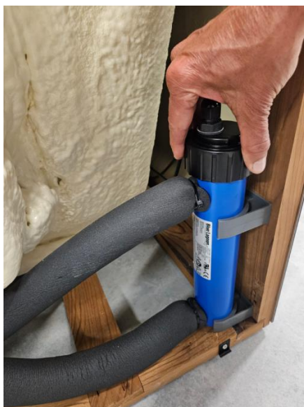
Fig. 10. Unscrew disinfector cover
