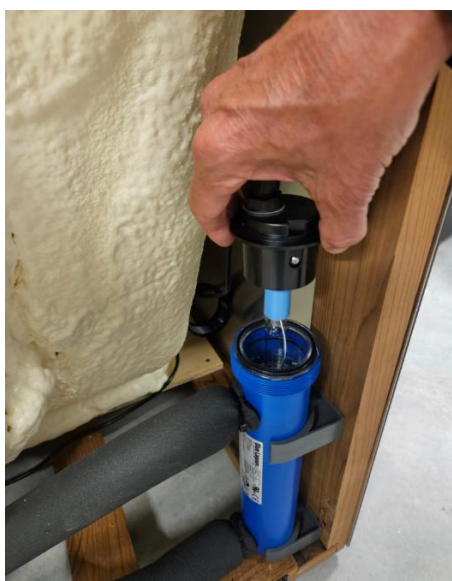
Fig. 11. Pull out/fit in UV-lamp
